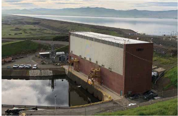
Figure 5. O'Neill Pumping Plant
