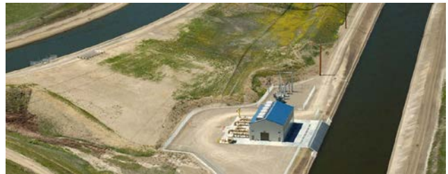
Figure 4. Intertie Pump Station located between the California Aqueduct and the Delta-Mendota Canals.
