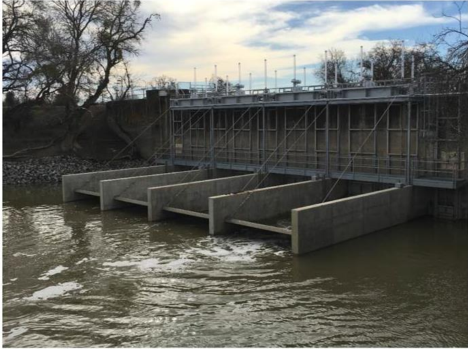
Figure 6. Knights Landing Outfall Gates (KLOG)
