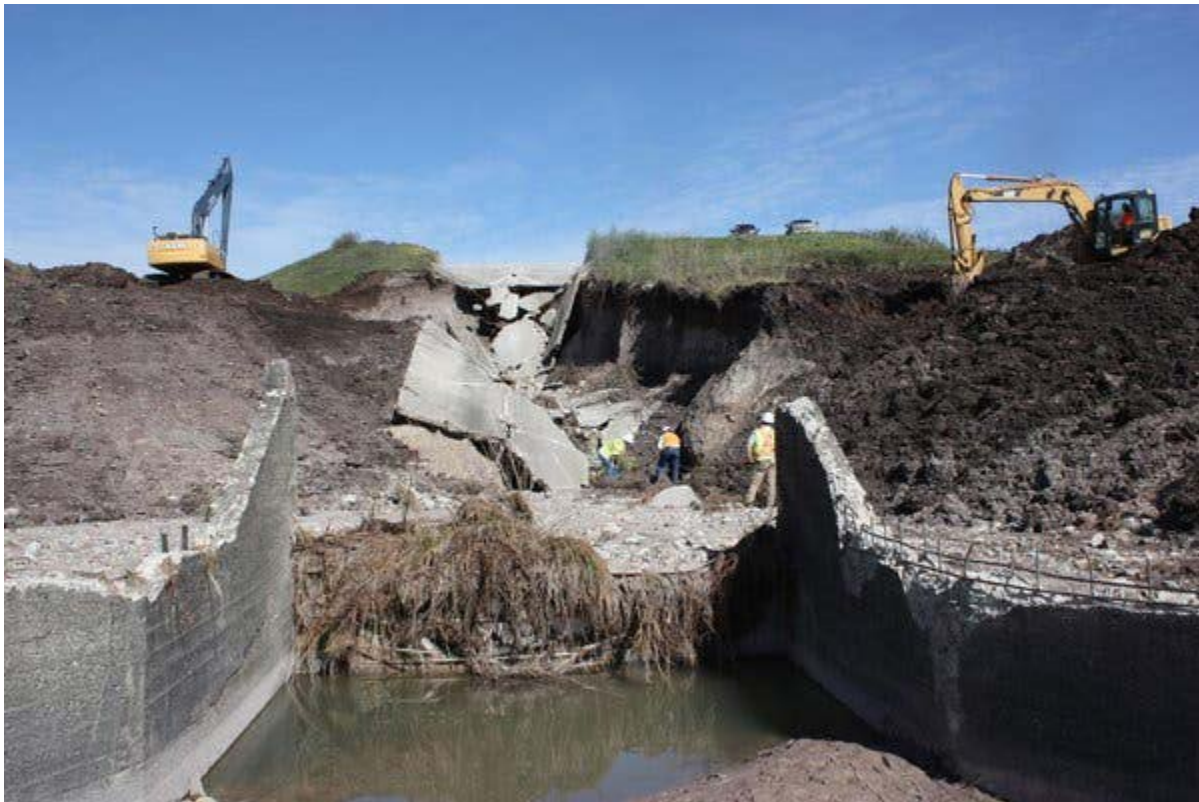
Collapsed Drop 5, Jim Robbins, Canal's Decay May Leave Montana Parched , N.Y. Times, June 16, 2020, at A12.
