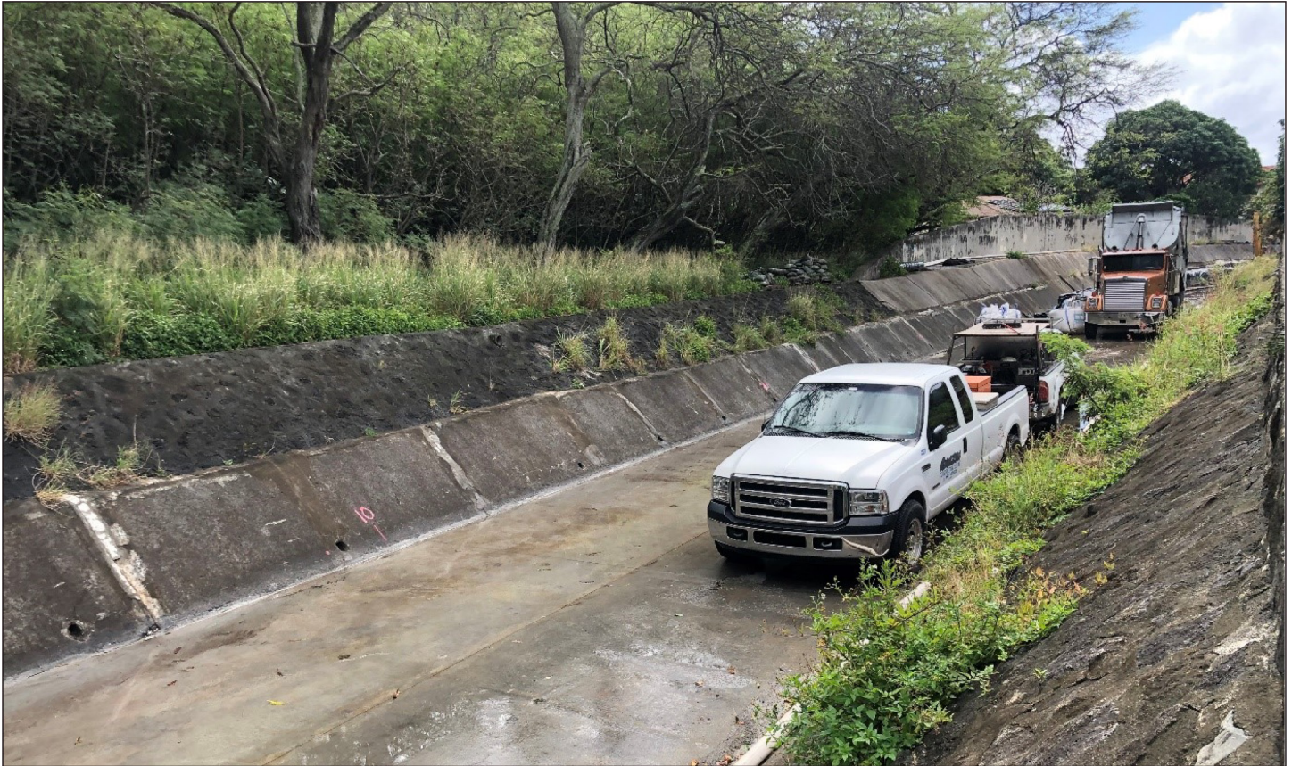
Figure 4: Public Assistance Project to Repair the Kuliouou Stream Flood Control Channel Damaged During Severe Flooding on the Island of Oahu, Hawaii, in April 2018
